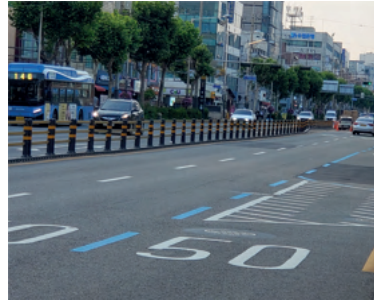
Jungwha station - Completed in 2021
