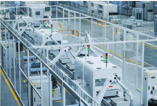
Receiving acoustic data generated during machine operation
